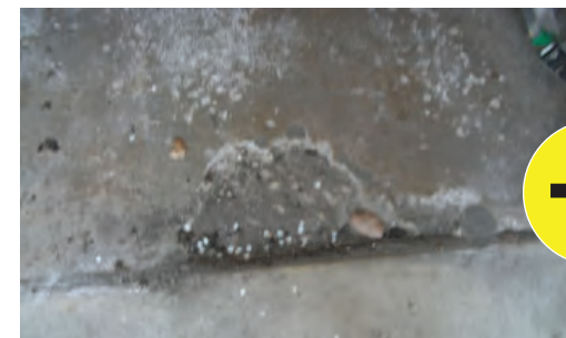
Joint Repair Before
