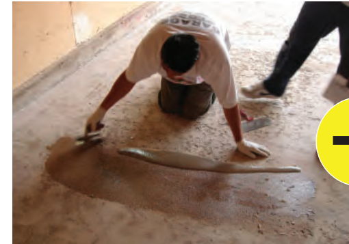
Repair with Trowel System
