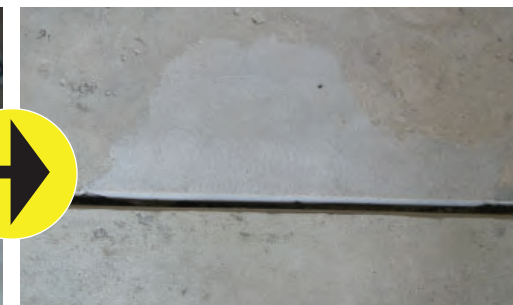
Joint Repair After
